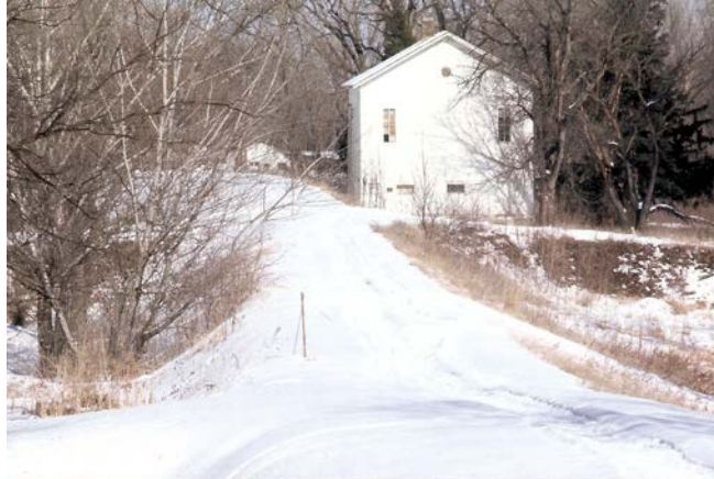
Mill/Masonic Lodge Building ca. 1980 (cotm)
