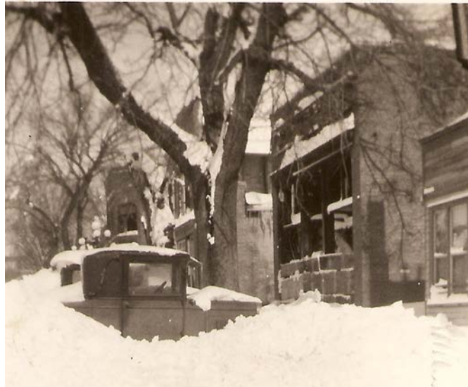
Wetter General Store after Fire, 1930s (unk)
