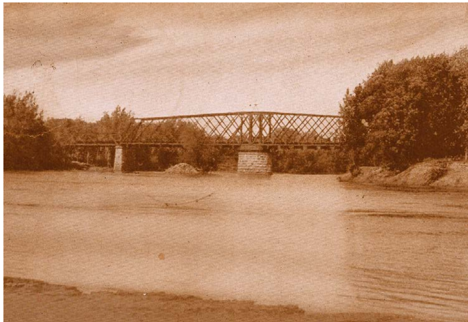
Mpls- St. Louis RR River Crossing Metal Truss Bridge, ca. 1909 (hp)
