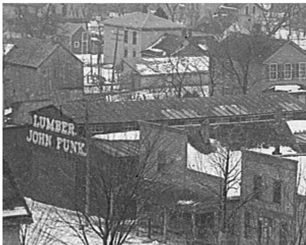
Funk Lumber Yard on Broadway in 1911, opposite the Hardware (cchs)
