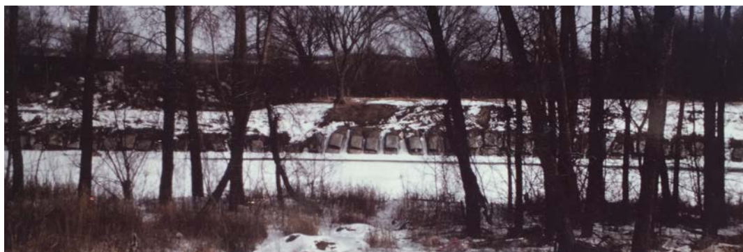
Strengthening the flood dike with junk cars, viewed from Scott County side, 1969 (cotm)
