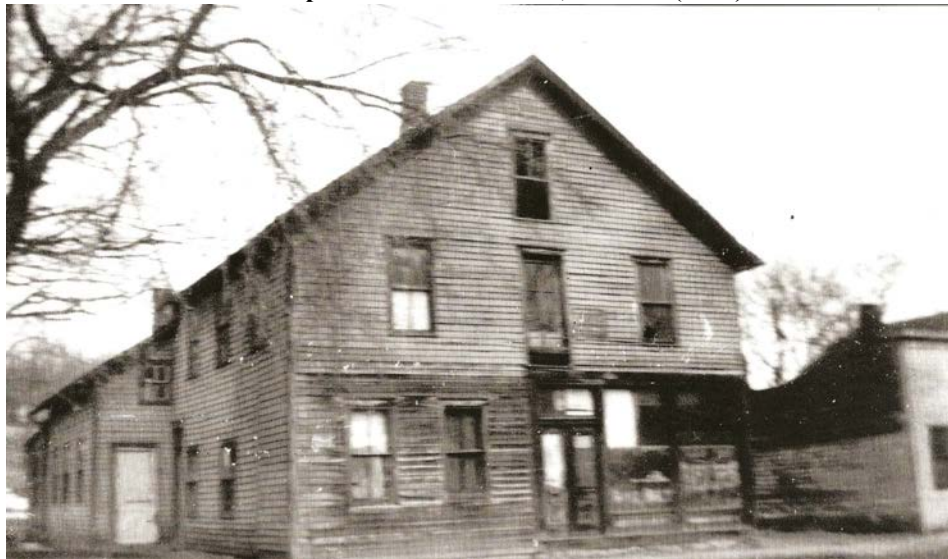
Shortly Before Demolition, the Minneapolis Hotel and Saloon, ca. 1940 (cotm)
