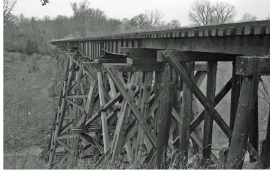
H & D Bridge over north Broadway, 1899 version (unk)
