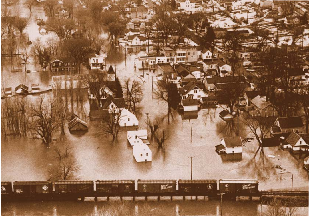
Aerial view, Carver flood, April 1965 (nai)
