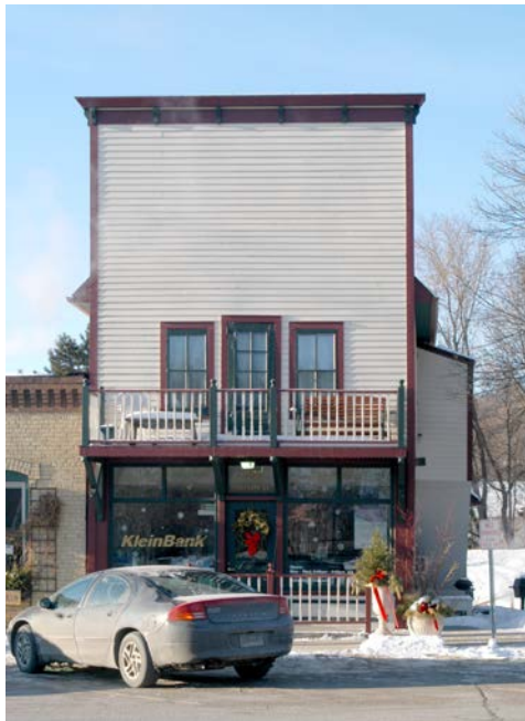
304 Broadway ca. 2010 after restoration
