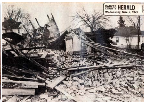
General Store Demolition, Nov. 1979 (ch)
