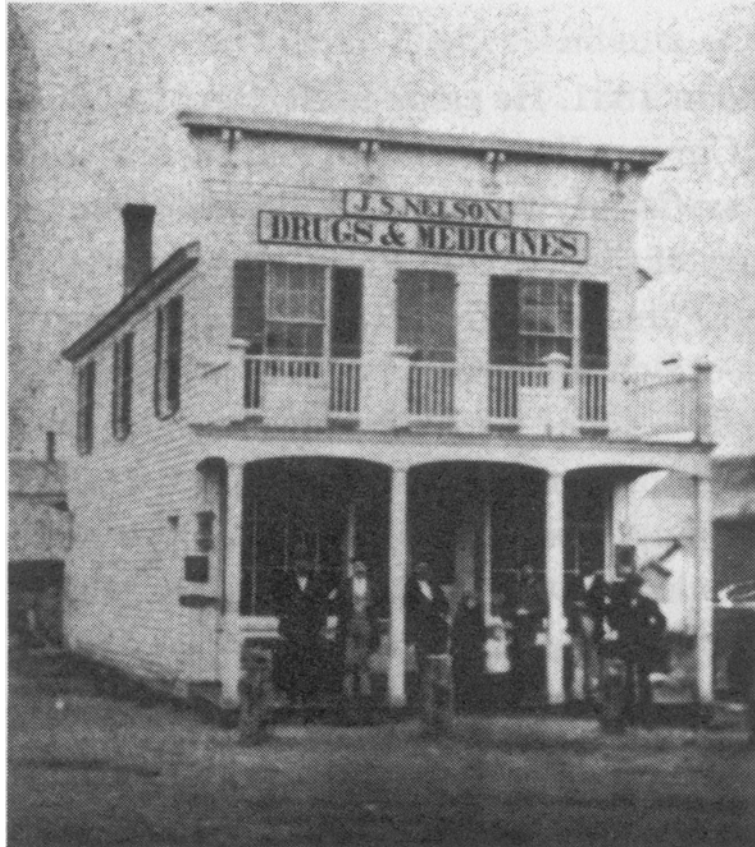
DuToit-Nelson-Brunius Building ca. 1875 (cotm)
