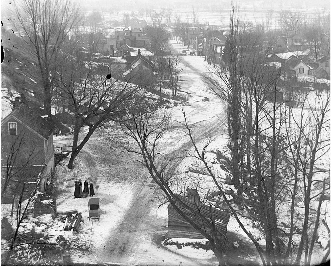
1911 View of Broadway Facing South from atop the H & D Railroad Bridge (cchs)
