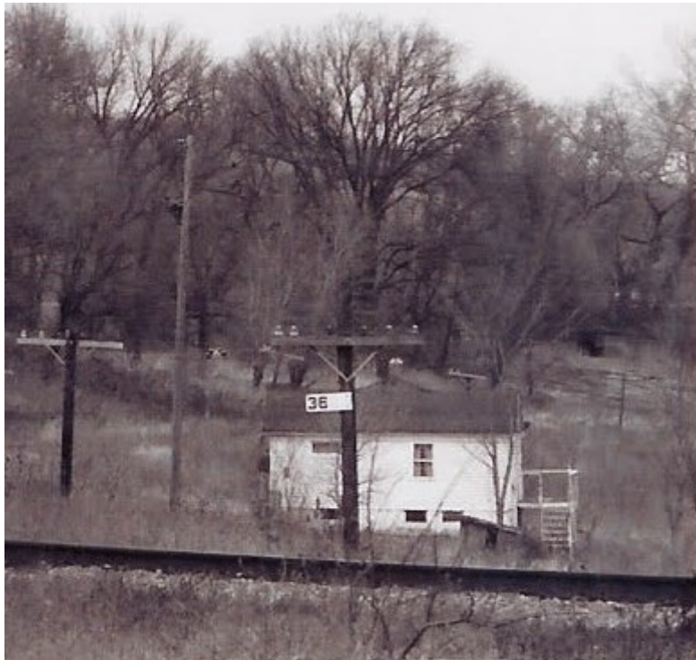
Former Fairgrounds Office Building (jm)
