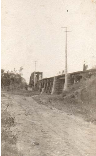
Road east of river crossing bridge that once ran down to Holmes' river bank elevator, cs. 1885 (unk)
