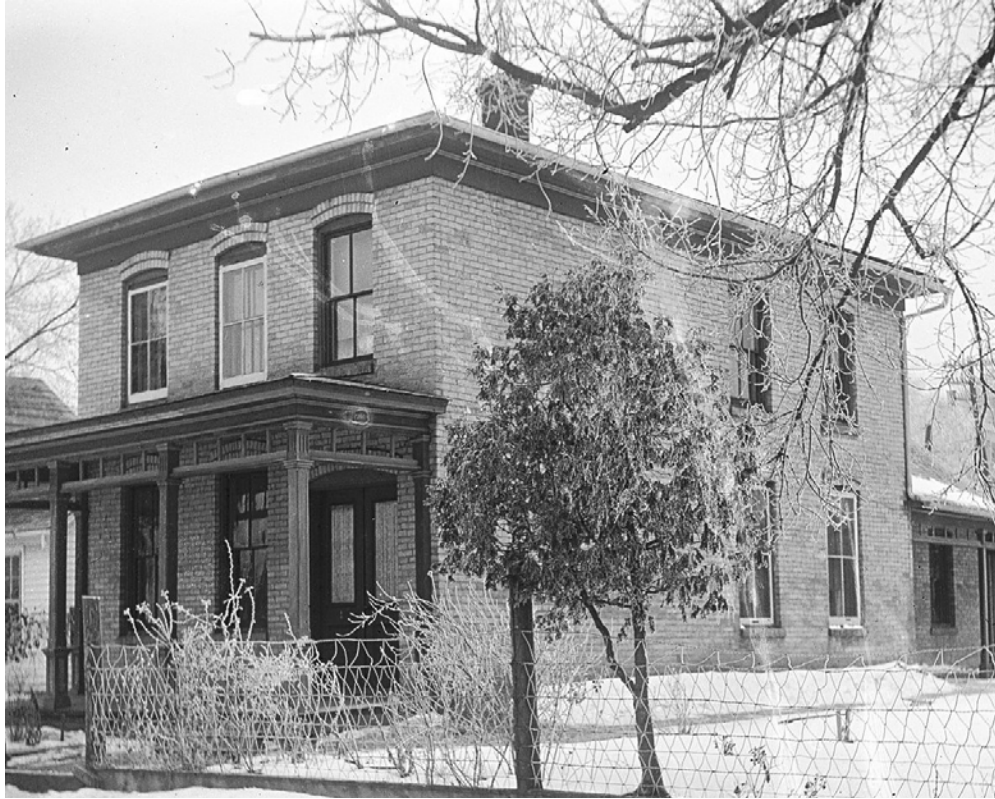
Johnson-Japs House (cchs)
