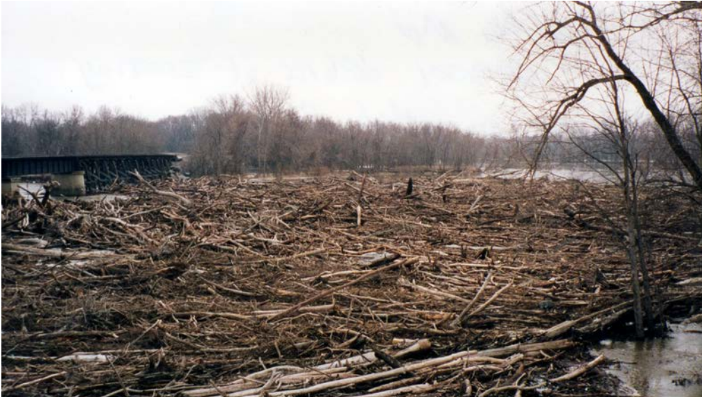
April, 2001 Flood Deadfalls Collected Against the RR River Crossing Bridge (unk)
