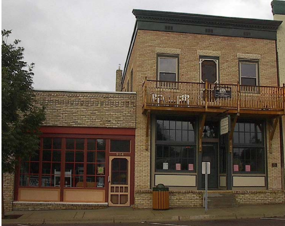
204 & 208 Broadway after restoration (jvw)
